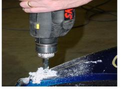
c. Drill the 1/8" hole for the lift the dot stud
